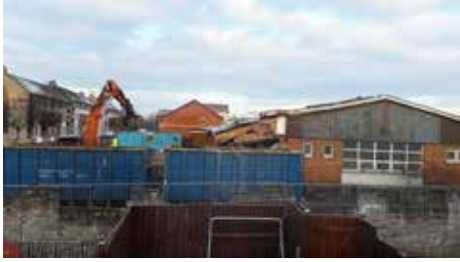
The old community centre going
