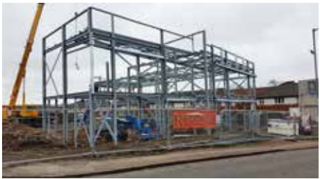
Work gets well under way on the new community centre
